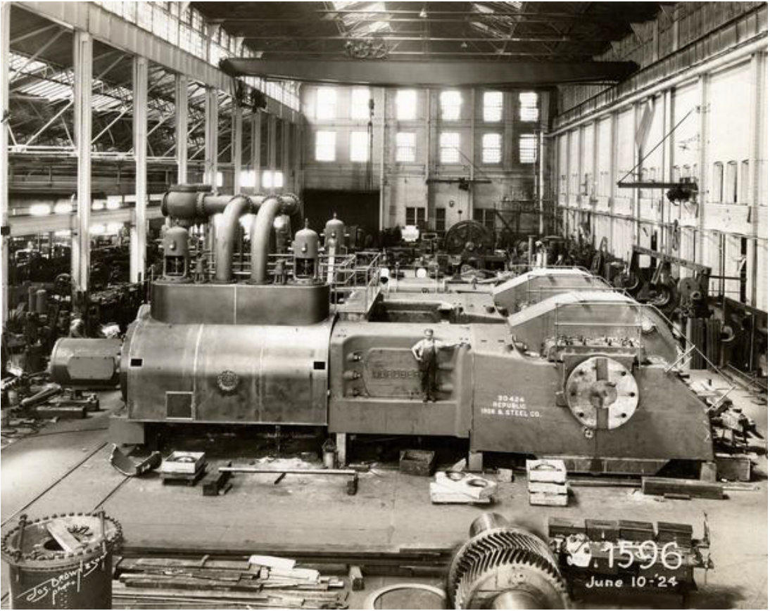
Worker stand on a Nordberg machine on the floor of what is likely a plant owned by Republic Iron & Steel Co.
